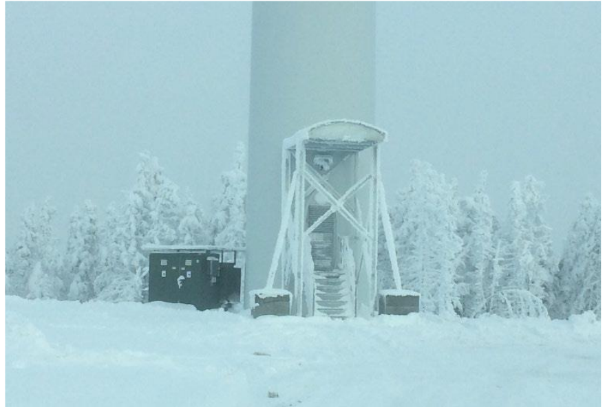
Figure 1 Permanent Ice Protection Device for Worker Access [1]
