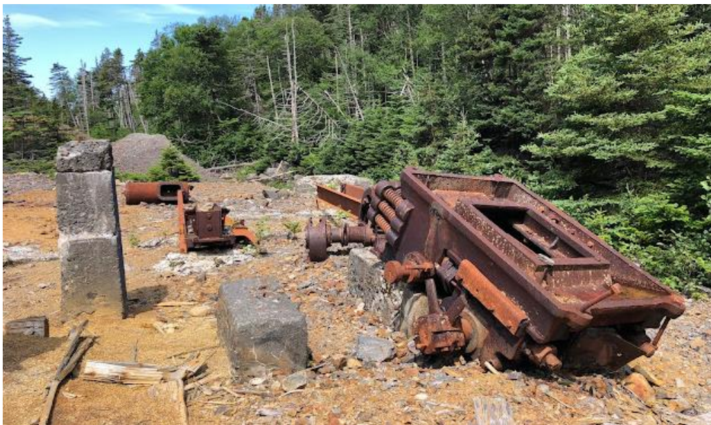
Figure F-3.3.1-5 View Northwest Along the South Shore of Broad Cove Brook Showing Dilapidated Mining Equipment at the Site of the Former Silver Cliff Mine Mill.
