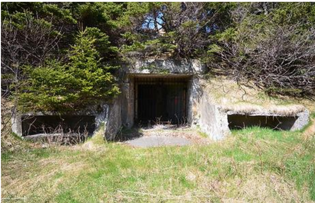
Figure F-3.6-1 Entrance to Underground Bunker at the 282 Coastal Defense Battery – a Designated Architectural Resource.
