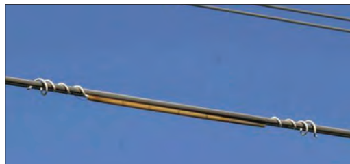
FIGURE 6.22: The Mace Bird Lite is a spiral device with a central fluorescent tube that is illuminated by the ambient electrical field.
