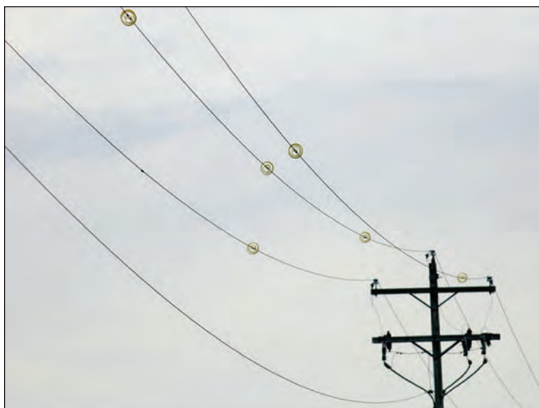
FIGURE 6.14: Swan-Flight™ Diversers installed on the phase conductors of a distribution line.
