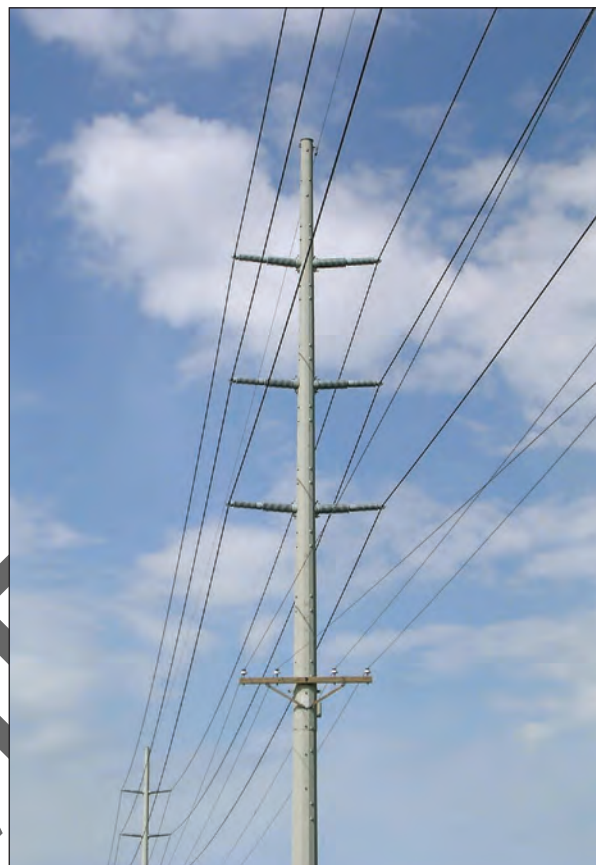
FIGURE 1.7: Distribution underbuild on a double-circuit transmission line.
