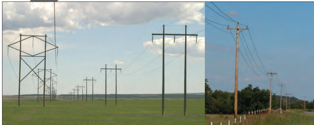
FIGURE 1.3: Transmission lines (left) and distribution lines (right).
