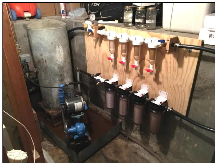
PHOTO 1: Particle Filter System (as observed by AECOM on 14-September-2017)
