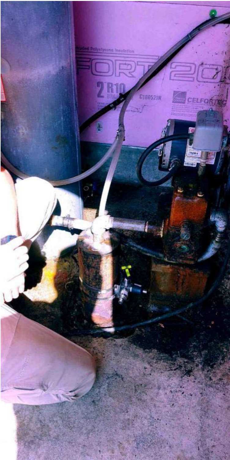
Photograph 2: Well 10 illustrating proximity of pump, hoses and tank to well casing.
