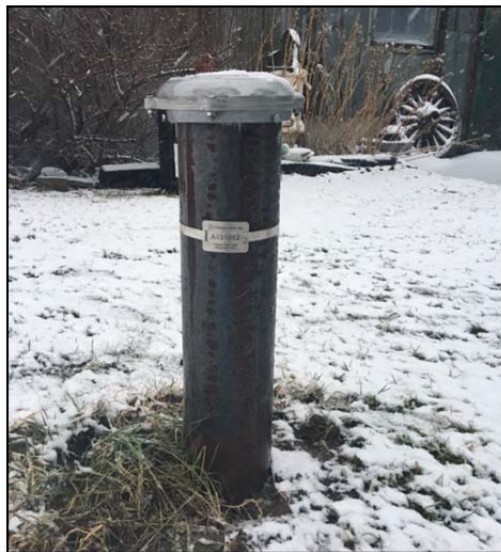
PHOTO 1: Drilled Water Well (as on 1-March-2018)
