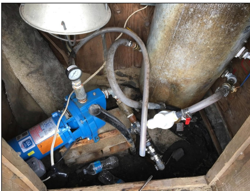
PHOTO 1: Well Pump & Particle Filter System (as observed on 4-October-2017)
