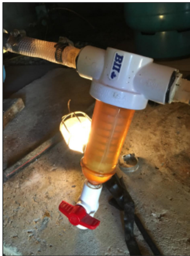
PHOTO 2: Visible iron fouling within sediment filter (as on 20-October-2017)
