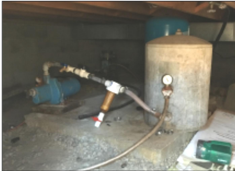
PHOTO 1: Well Pump & Particle Filter System (as observed on 20-October-2017)
