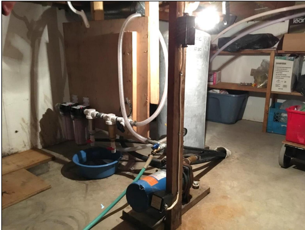
PHOTO 1: Well Pump & Particle Filter System (as observed by AECOM on 18-September-2017)
