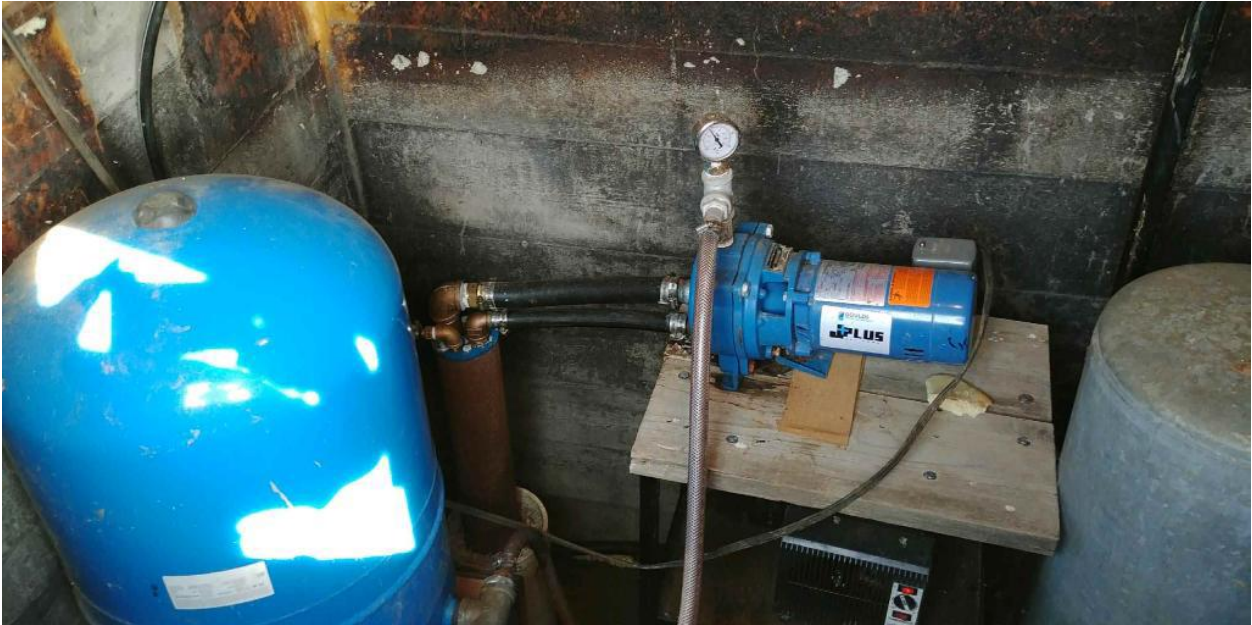
Photograph 1: Well 6 illustrating proximity of pump, hoses and tank to well casing.
