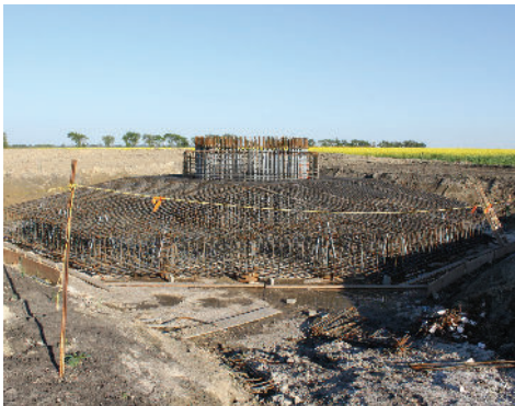
Foundation rebar
