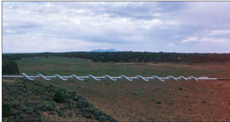
FIGURE 6.10: Spiral vibration dampers act to reduce line vibration, and they also make power lines more visible to birds.
