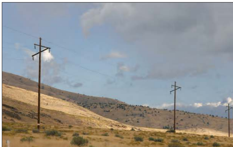
FIGURE 4.19: Orientation of power lines parallel to ridges or narrow, low altitude flyways presents a lower risk of collision than perpendicular orientation.
