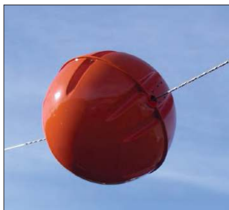
FIGURE 6.8: Aerial marker spheres, also known as aviation balls, were designed to make power lines more visible to aircraft operators.
