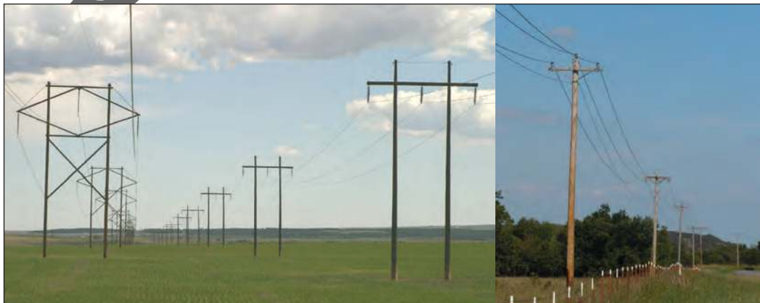
FIGURE 1.3: Transmission lines (left) and distribution lines (right).
