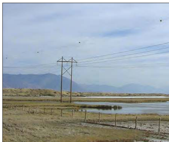
FIGURE 6.9: Aerial marker spheres in use on a power line above a wetland habitat.
