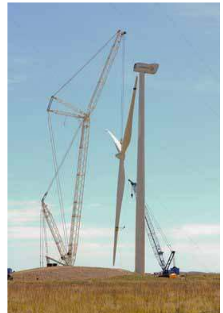
Towers are being lifted as work continues on the 2 MW Gamesa wind turbine that is being installed at the NWTCC. Credit: NREL
