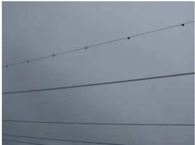
Figure 6.5. Preformed Swan Flight Diverter installed on overhead lines with alternating Power Line Sentry Bird Flight Diverter.
