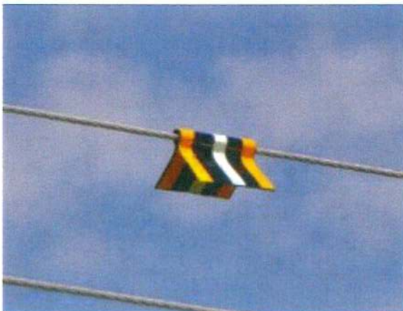
Figure 6.2. Power Line Sentry Bird Flight Diverter.
