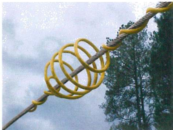
Figure 6.4. Preformed Swan Flight Diverter.
