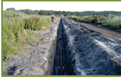
Typical Collector Line Trench
