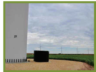
Typical Pad-mounted Transformer
