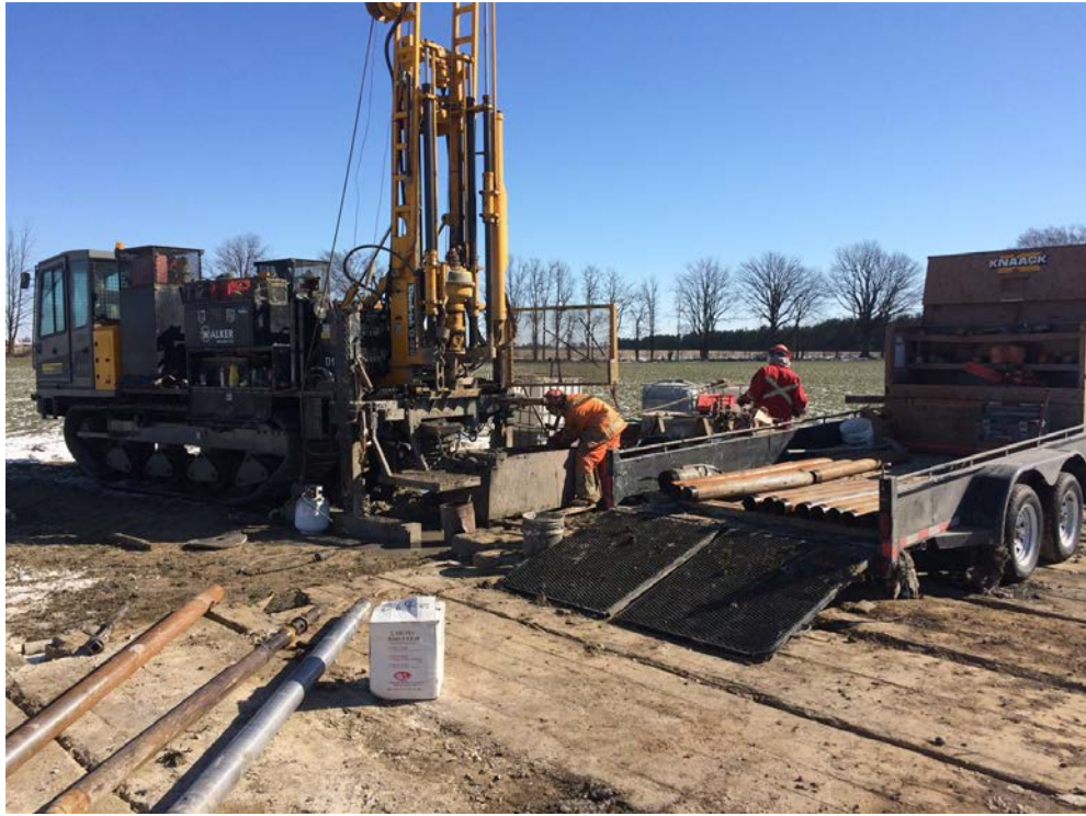
Photograph 13: Drilling for borehole installation of accelerometers at T42 site.
