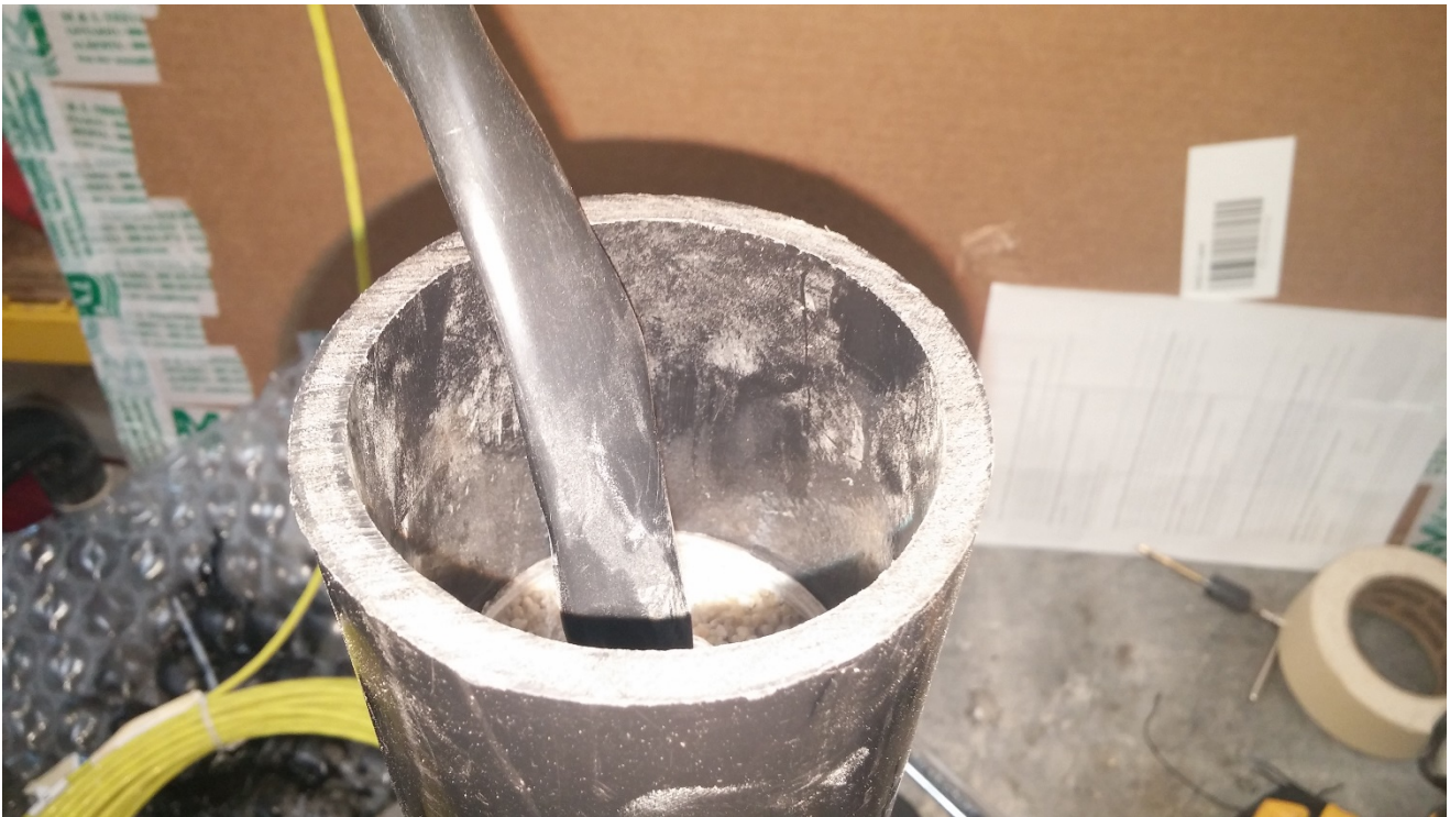
Photograph 9: Top of protective housing, showing infilling with sand and clear plastic top cover (later sealed against water intrusion).
