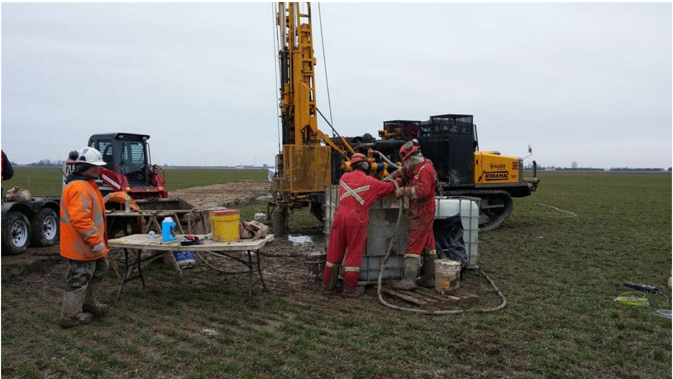
Photograph 17: Installation of accelerometers in borehole at T42 site.
