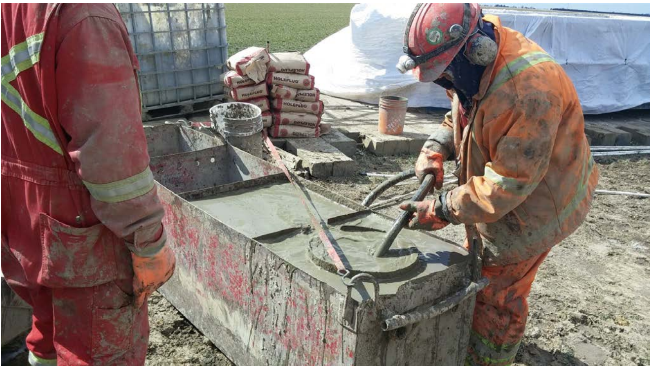
Photograph 18: Bucket immersed in grout for measuring down-hole grout quantities for coupling accelerometer housing to soil or rock in bottom of boreholes at T42 site.
