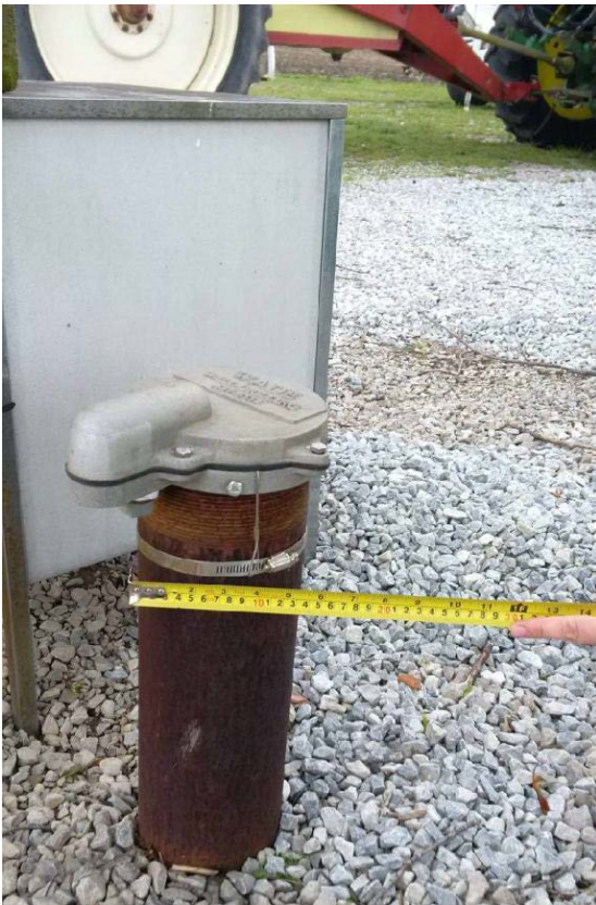
Photograph 33: Well #3 casing and well lid conditions (note band/hose clamp and wire leading into well through gasket).
