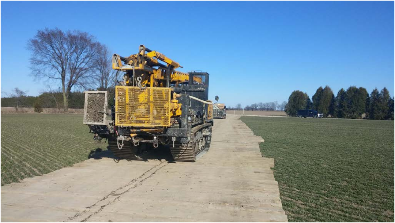
Photograph 19: Drill rig tracking toward Claymore Line on timber mats at T42 site.
