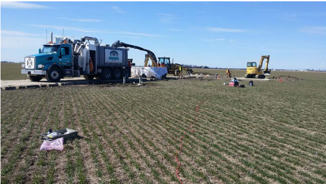
Photograph 22: Vacuum truck operating at T42 site to remove cuttings and fluids after completion of installation and during baseline instrument readings.
