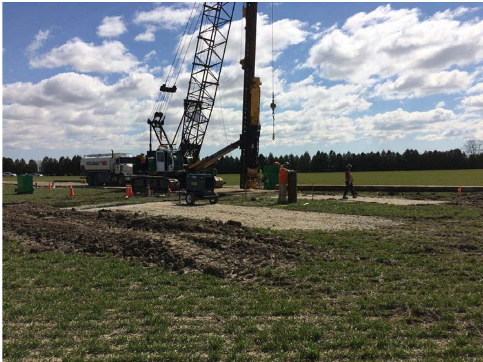
Photograph 25: Pile driving on March 29, 2017 showing first pile section driven, second pile section on ground awaiting lifting and welding.
