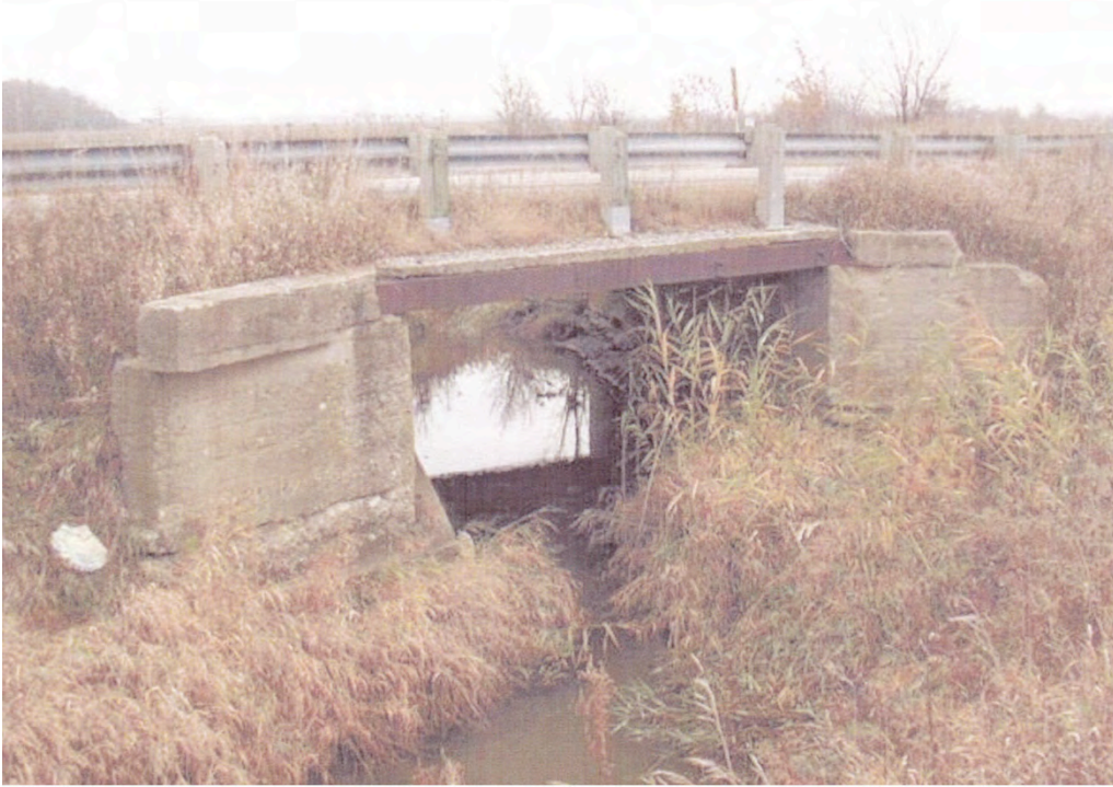
Figure 24: The old Horne Drain (1945) had a concrete deck supported by conventional steel girders. (This construct replaced an earlier culvert built in 1915. (Municipaltools.com, 2012))
