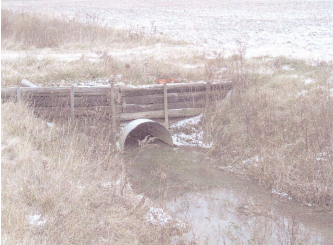
Figure 26: Rail ties and angle irons used for culvert on the south side of 8 th Line west of Wellwood.
