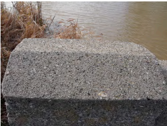
Figure 58: Cap of concrete abutment forming part of the marina bridge
