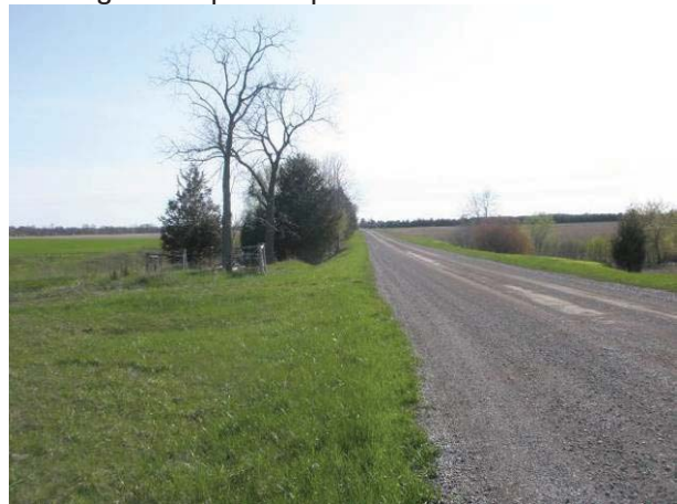
Field Plate 53.50: View southwest along Collector Line on New Scotland Line at roadbed, fill slope and ditching – no potential.
