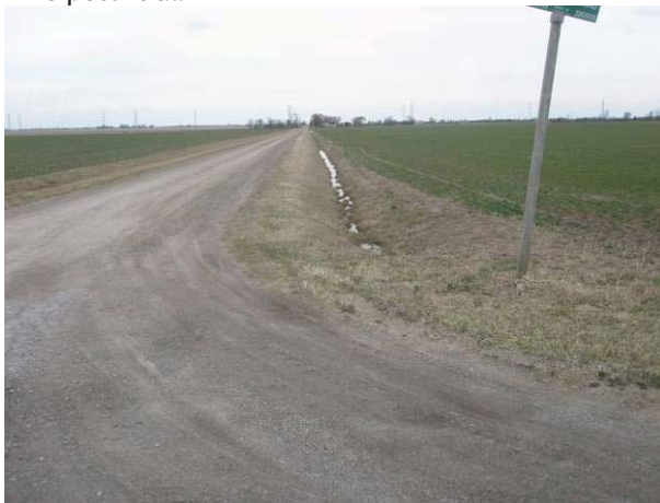
Field Plate 51.9: View northwest along Collector Line on Cooper Road, east side, at ditching and disturbed roadbed with no potential.
