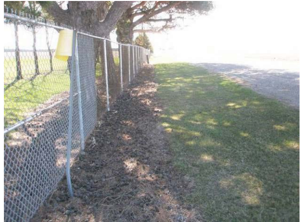
Field Plate 52.4: View southeast along Collector Line Bloomfield Road, east side, at disturbed roadbed and shoulder – no potential.
