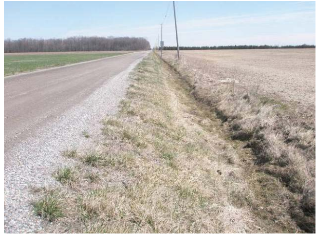
Field Plate 52.8: View northeast along Collector Line on Tenth Line, east side, at disturbed roadbed and ditch in ROW – no potential.
