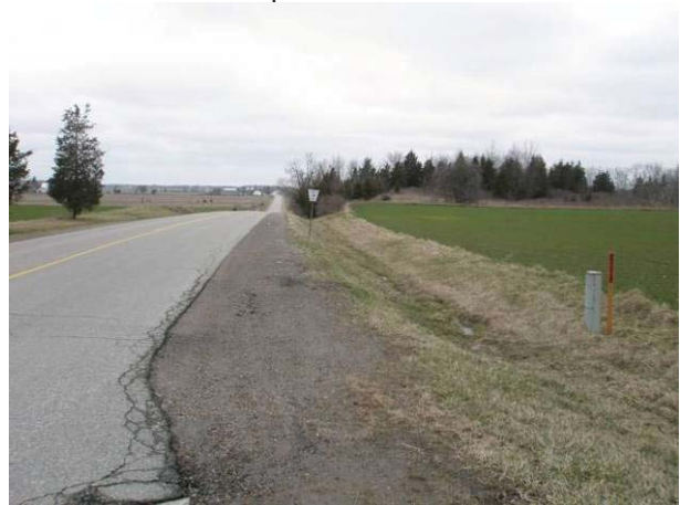
Field Plate 53.6: View northwest along Collector Line on Mull Road at ditching and buried utilities in ROW – no potential.
