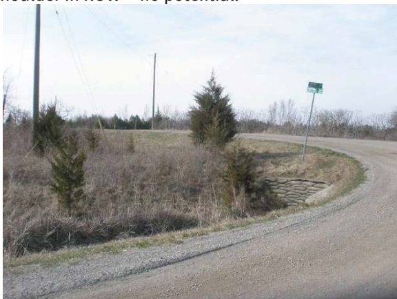
Field Plate 52.35: View northeast along Collector Line on Drury Line at ditch in ROW – no potential.
