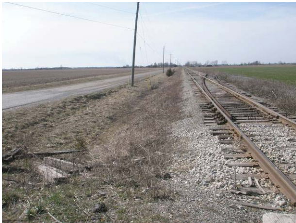
Field Plate 52.31: View northwest along Fargo Road from Drury Line at disturbed ROW between roadway and rail line – no potential.
