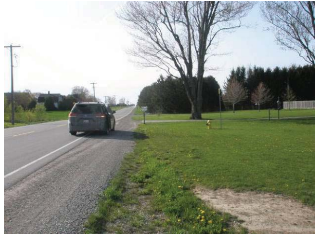
Field Plate 53.52: View northwest along Collector Line on Kent Bridge Road at disturbed roadbed, shoulder and graded residential lawn with buried utilities – no potential.
