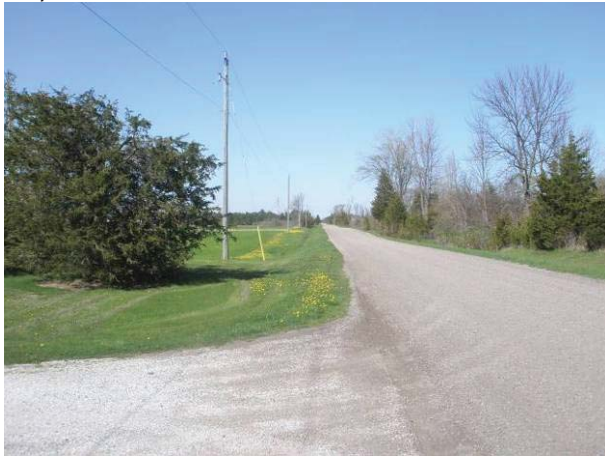
Field Plate 53.41: View northeast along Collector Line on Ed's Line at raised roadbed and ditching in disturbed ROW.
