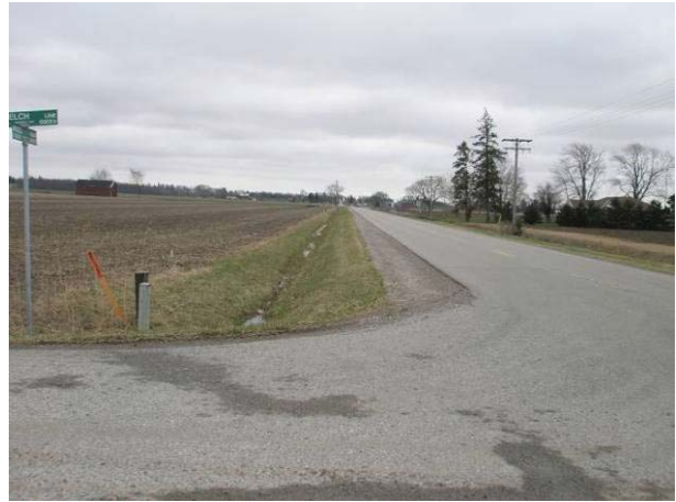
Field Plate 53.4: View southeast along Collector Line on Mull Road at raised roadbed, ditching and buried utilities in ROW – no potential.
