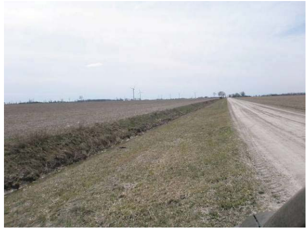
Field Plate 51.38: View south along Collector Line on Oak Road at Middle Line at raised roadbed and wide shoulder to ditch in ROW – no potential.
