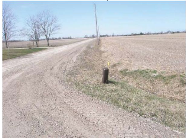
Field Plate 51.40: View west along Collector Line on Gray Line, north side, at droadbed, shallow ditching and buried telephone line – no potential in ROW.
