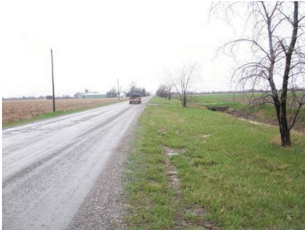
Field Plate 53.9: View northwest along Collector Line on Welch Line, east side, at area with potential between roadway and creek that was tested at 5 m.
