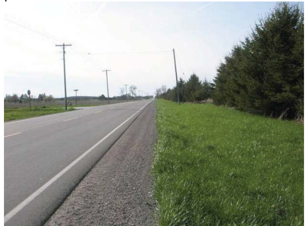
Field Plate 53.54: View northwest along Collector Line on Kent Bridge Road at disturbed ROW with no potential.
