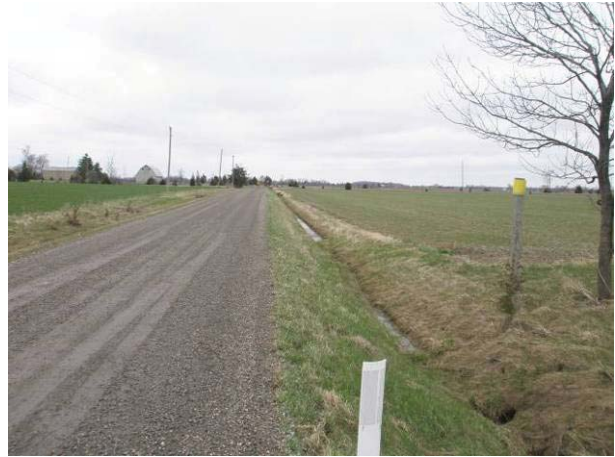
Field Plate 52.56: View northeast along Collector Line on Knights Line towards Base Road at disturbed ROW with no potential.
