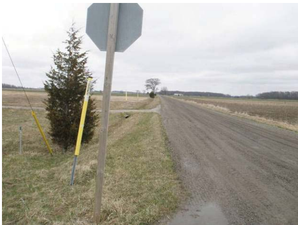
Field Plate 53.1: View northeast along Collector Line on Welch Line at raised roadbed and ditch – no pot'l.
