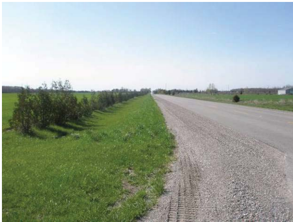
Field Plate 53.43: View northwest along Collector Line on Kent Bridge Road at wide ditching – no potential.
