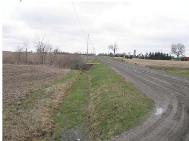
Field Plate 52.60: View southwest along Collector Line on Burk Line at raised roadbed and ditching in ROW.
