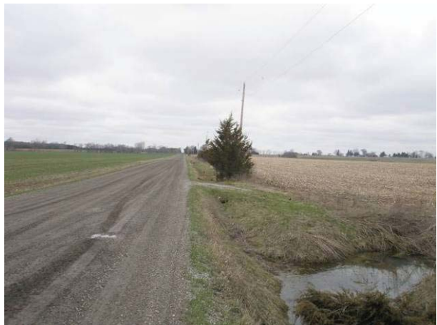
Field Plate 53.20: View northwest along Collector Line on Mull Road at disturbed roadbed and ditching – no potential.
