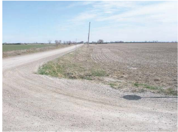
Field Plate 51.32: View northeast along Collector Line on Morris Line, south side, at raised roadbed and shallow ditching in ROW – no potential.
