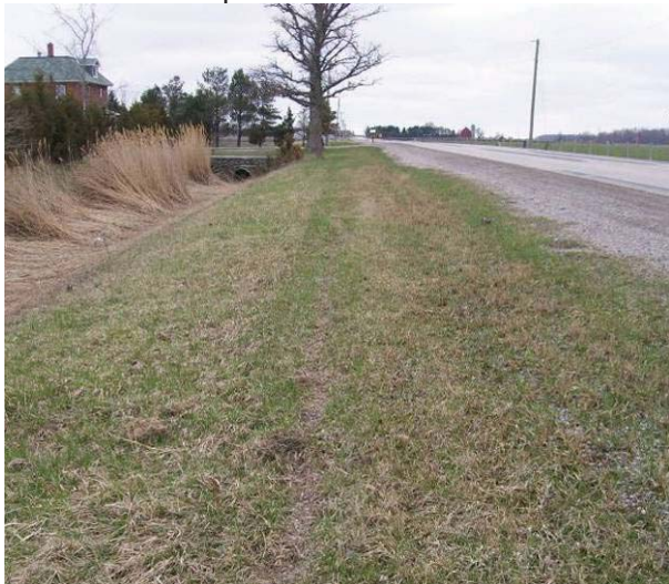
Field Plate 52.33: View southwest along Collector Line on Drury Line, south side, at disturbed roadbed and shoulder in ROW – no potential.
