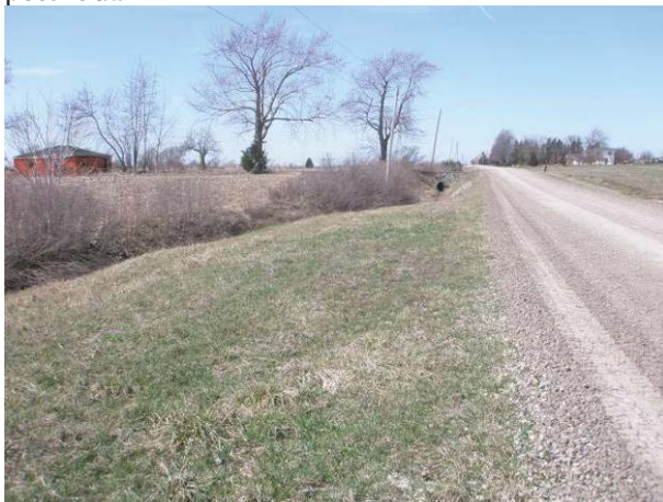
Field Plate 51.41: View west along Collector Line on Gray Line, south side, at disturbed ROW with no potential.
