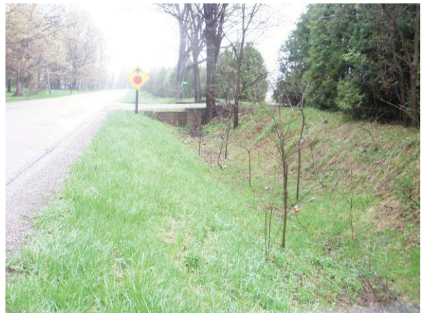
Field Plate 52.24: View northeast along Collector Line on Doyle Line, south side, towards Garden Road.
