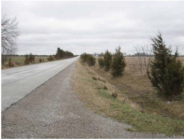
Field Plate 52.49CL: View southeast along Collector Line on Harwich Road at raised roadbed and ditching.
