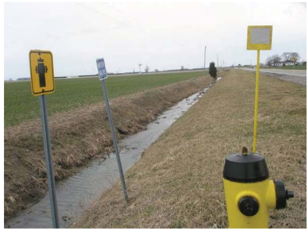
Field Plate 51.8: View southwest along Collector Line on Port Road at raised roadbed, ditching and buried utilities in ROW – no potential.
