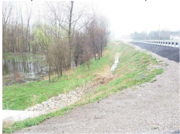
Field Plate 52.28: View southwest along Collector Line on Boundary Line at disturbed roadbed and deep ditch – no potential.
