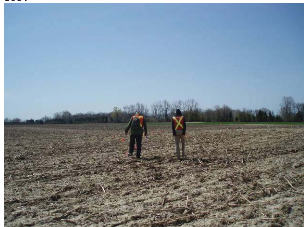
Field Plate 48.6: View south across TPA-103 turbine pad and access road.
