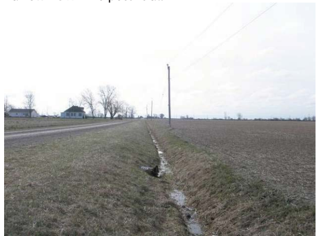
Field Plate 51.28: View southeast along Collector Line on Cooper Road, west side, at raised roadbed and ditching – no potential.
