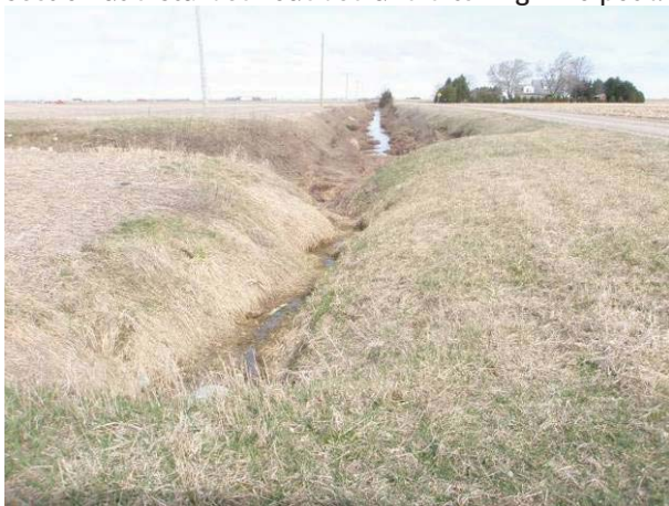
Field Plate 51.29: View southwest along Collector Line on Gray Line, south side, at wide ditching and raised roadbed with no potential.
