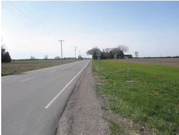
Field Plate 53.45: View northwest along Collector Line on Kent Bridge Road at disturbed roadbed, shoulder and ditching.
