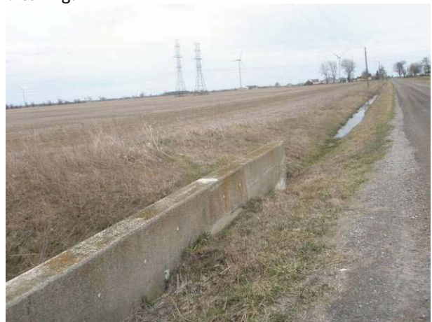
Field Plate 51.16: View southeast along Collector Line on Wellwood Road east side, at roadbed and ditching – no potential.
