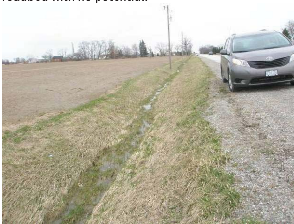
Field Plate 51.11 View southwest along Collector Line on Port Road, south side, at disturbed ROW – no potential.
