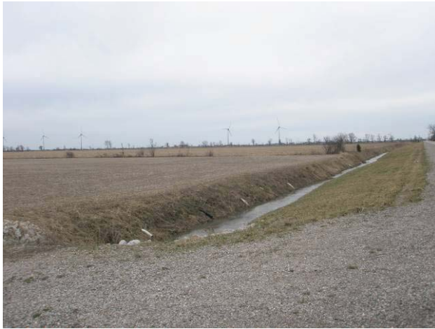
Field Plate 51.13: View southwest along Collector Line on Eighth Line, south side, at disturbed ROW with no potential.
