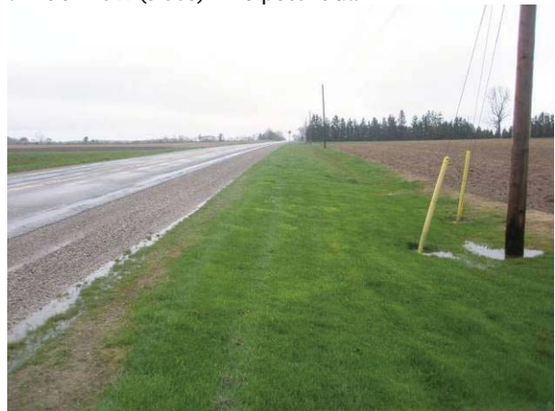
Field Plate 53.32: View southeast along Collector Line on Kent Bridge Road at raised roadbed and gentle fill slope in ROW – no potential.
