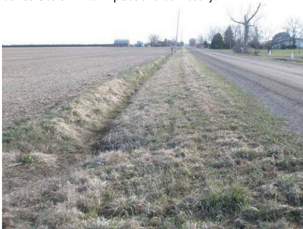
Field Plate 51.51: View northeast along Collector Line on 7 th Line West, north side, at raised roadbed and ditch in ROW – no potential.
