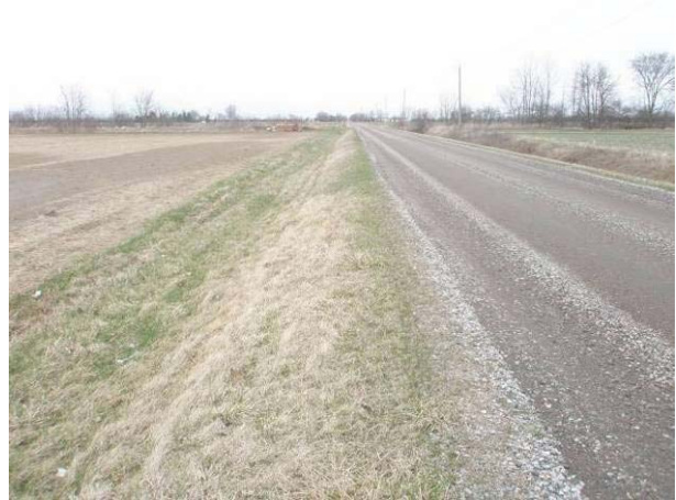
Field Plate 51.22: View northeast along Collector Line on Seventh Line, north side.
