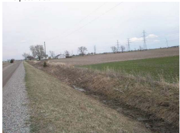
Field Plate 51.18: View northeast along Collector Line on Seventh Line, south side, at disturbed ROW.
