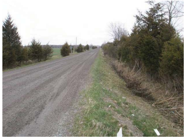
Field Plate 52.50: View southwest along Collector Line on Harwich Road at roadbed and ditching with no potential.
