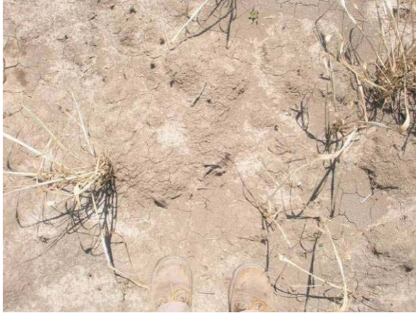
Field Plate 28.3: View of typical ground conditions at access road to TPA-038.
