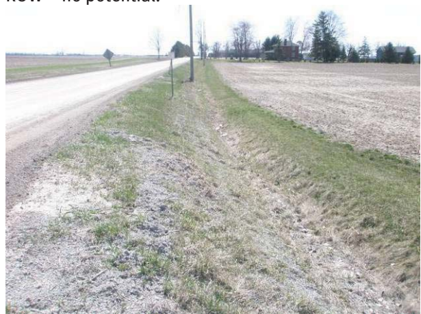
Field Plate 52.18: View southwest along Collector Line on Horton Line, north side, at disturbed ROW – no potential.
