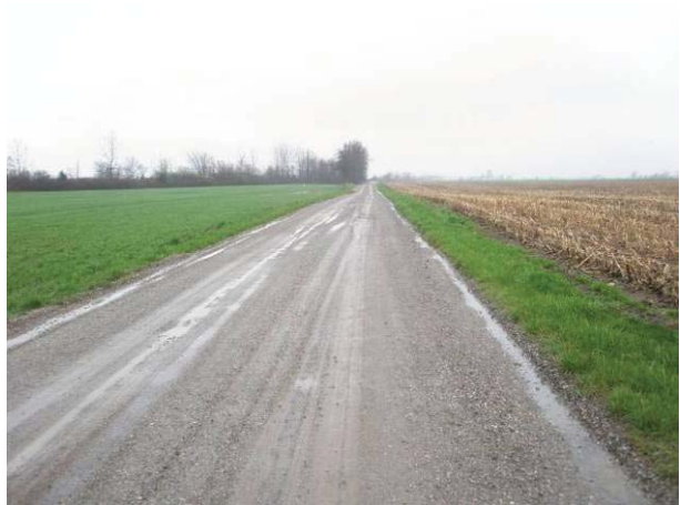
Field Plate 53.16: View southwest along Collector Line on Coffell Line at disturbed roadbed and shoulder in narrow ROW – no potential.
