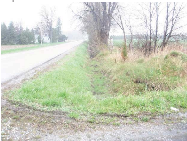
Field Plate 52.23: View northeast along Collection Line on Doyle Line, south side, from Fargo Road at disturbed ROW – no potential.
