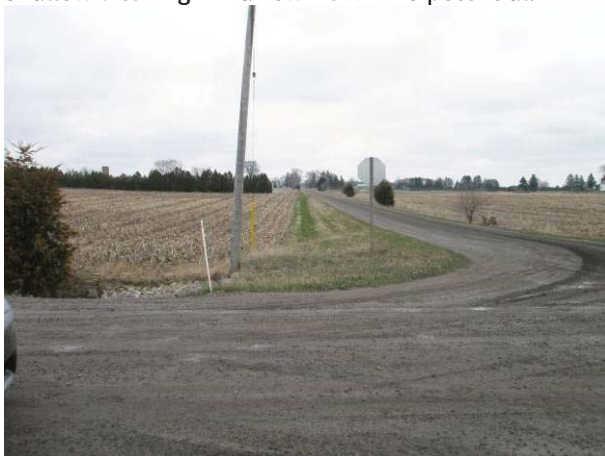
Field Plate 53.19: View northeast along Collector Line on Brush Line at raised roadbed and ditching to limit of ROW – no potential.
