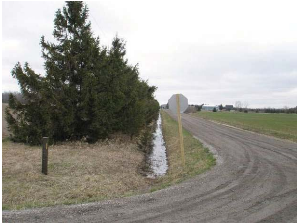
Field Plate 53.21: View southwest along Collector Line Stefina Line at ditching to limit of ROW – no potential.
