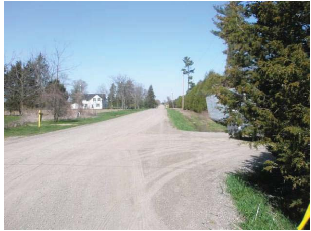
Field Plate 53.34: View northeast along Collector Line on Ed's Line at raised roadbed and ditching in ROW – no potential.
