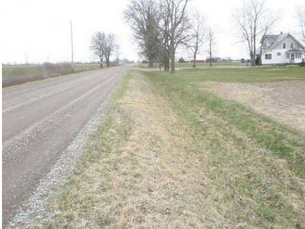
Field Plate 51.21: View southwest along Collector Line on Seventh Line, north side, at raised roadbed – no potential.
