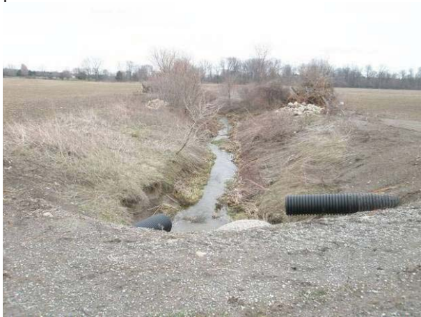
Field Plate 53.25: View west across Collector Line from Stefina Line at channelized stream.
