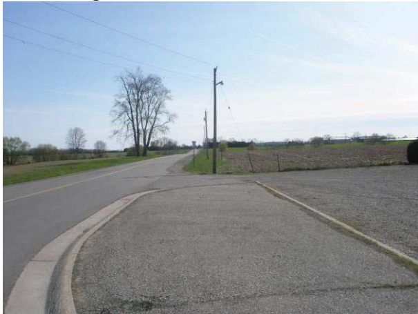
Field Plate 53.47CL: View southwest along Collector Line on New Scotland Line at disturbed roadbed and ditching in narrow ROW – no potential.
