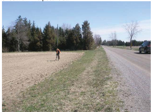
Field Plate 52.6: View northeast along Collector Line on Ninth Line, north side, at disturbed roadbed and fill in ROW – no potential.
