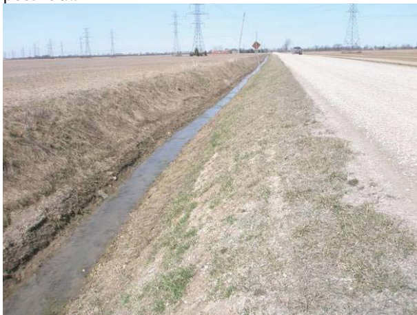
Field Plate 51.35: View northwest along Collector Line on Pollard Road from Morris Line, south side, at disturbed roadbed and wide ditching with no pot'l.
