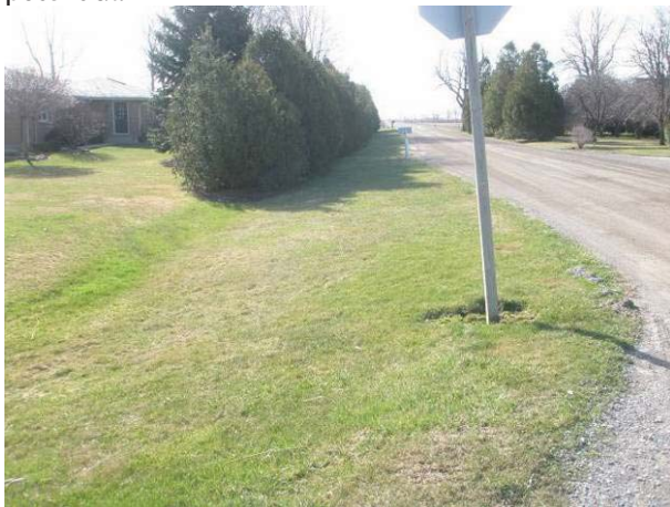
Field Plate 51.57: View southeast along Collector Line on Dillon Line, east side, at raised roadbed and fill slope to limit of ROW – no potential.
