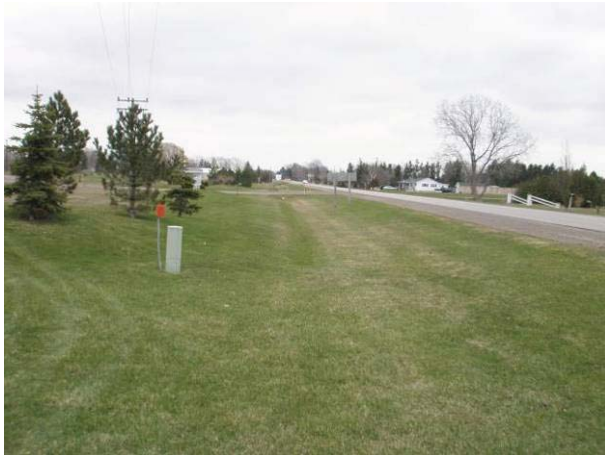
Field Plate 53.27: View southeast along Collector Line on Chatham Street at raised roadbed, wide ditching and buried utilities in ROW – no potential.
