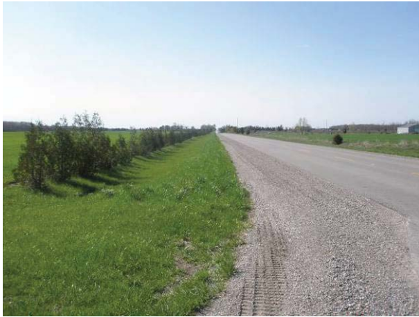
Field Plate 53.39: View northeast along Collector Line on Ed's Line at raised roadbed and fill slope in ROW – no potential.
