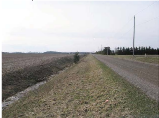
Field Plate 52.40: View northwest along Collector Line on Huffman Road, west side, at disturbed ROW with no potential.
