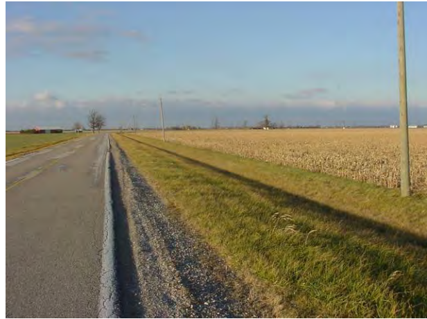
Plate 14: View to north along County Road 14 (Port Road). Elevated roadbed & roadside ditching in level terrain.
