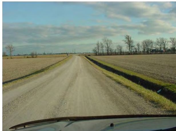
Plate 16: View to southeast along McKinlay Road from rail crossing. Note level terrain, elevated roadbed, road side ditching and field drain exit.
